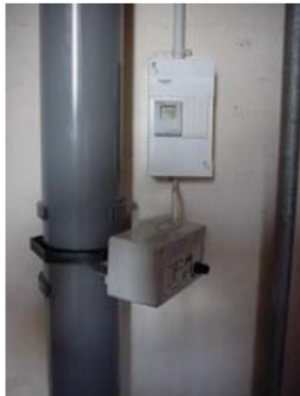
Fan and variable frequency controls
