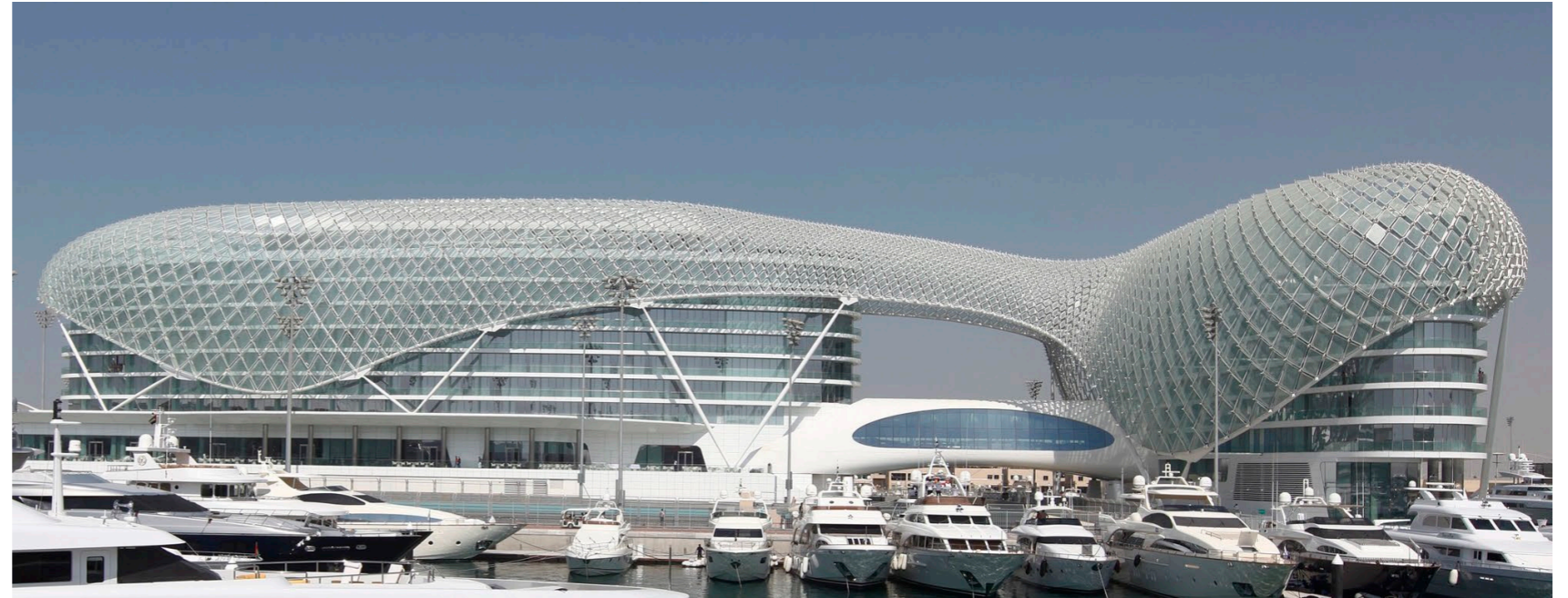
Yas Hotel Abu Dhabi, Arch. Asymptote Architecture Quelle: ArchDaily
