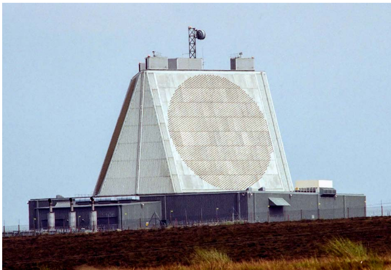
Figure 3 BMEWS solid-state phased-array radar at RAF Fylingdales, UK. ( https://commons.wikimedia.org/wiki/File:Radar_RAF_Fylingdales.jpg )
