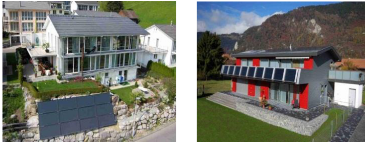
Fig. 5. On-site generation (pictures [2]).
