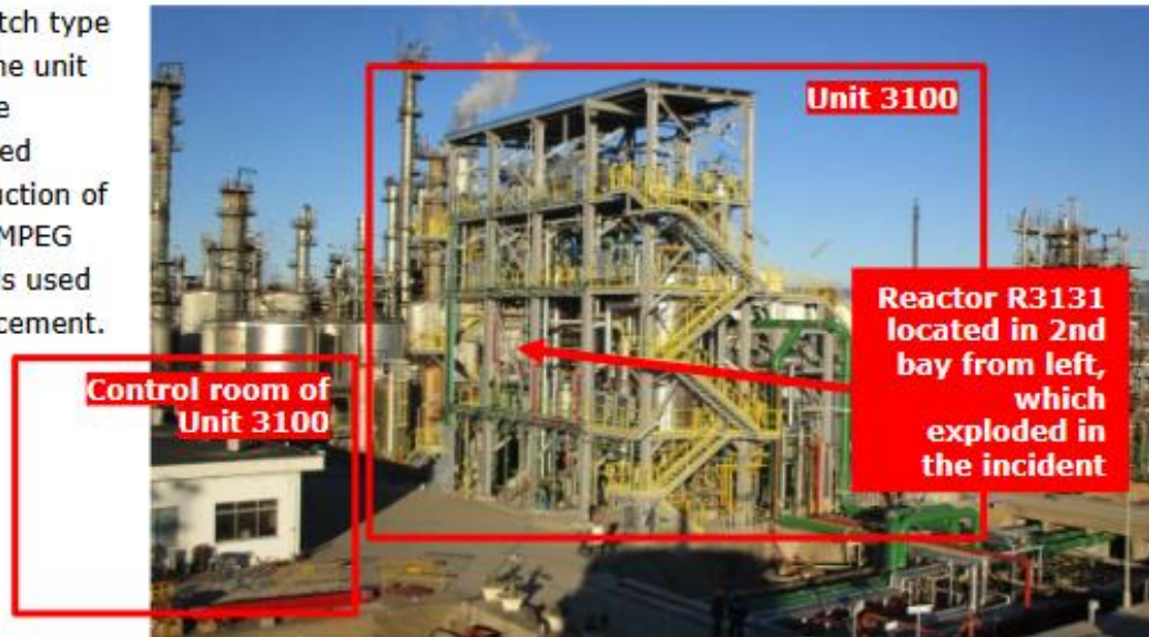
Figure 3-2: Unit 3100 prior to the explosion
