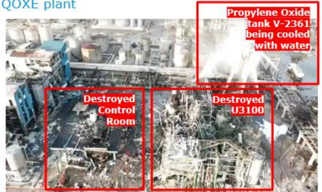
Figure 3-5: Excerpt from video showing the destroyed U3100 and surrounding facilities
