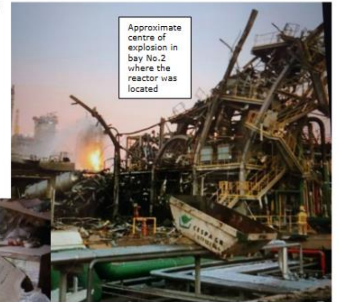
Figure 3-3: U3100 directly after the explosion
