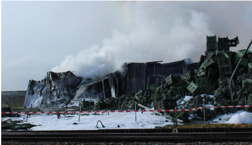
Figure 2: Photo shows the extent of the major fire at Tobi Seeobst in Egnach TG [31].
