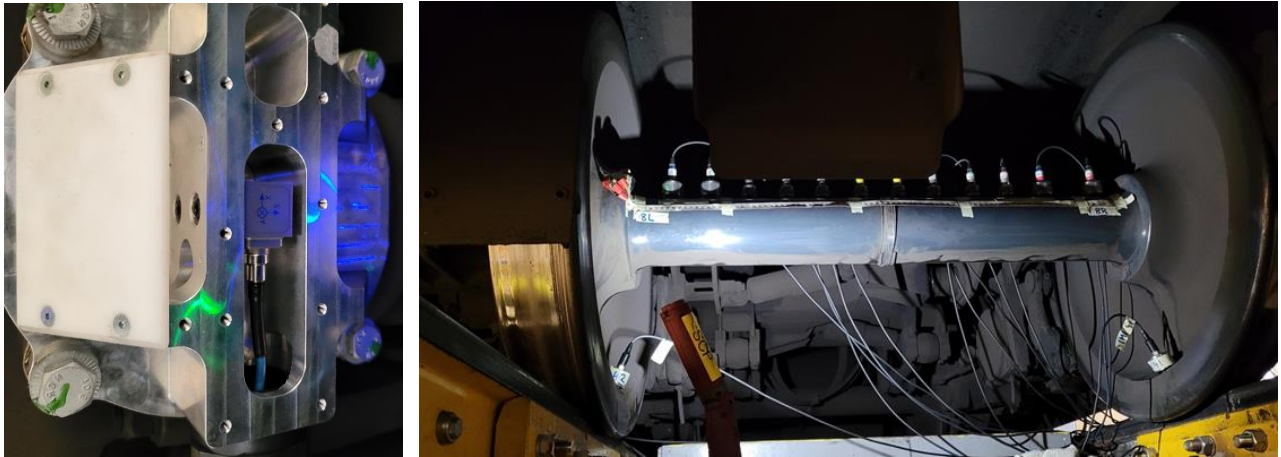
Fig.4 Schematic drawing of a railway axel and mounted accelerometer sensor(s) and example of mounted sensors on axel end (bottom left) and on the axel (bottom right).
