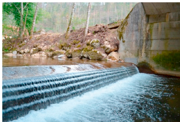
Fig. 9. Crayfish barrier in the Lützel with aluminium plates attached on to the pillars of the bridge.
