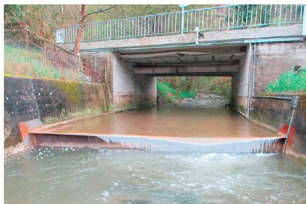
Fig. 8. Crayfish barrier with overhanging lip in the Etzgerbach .
