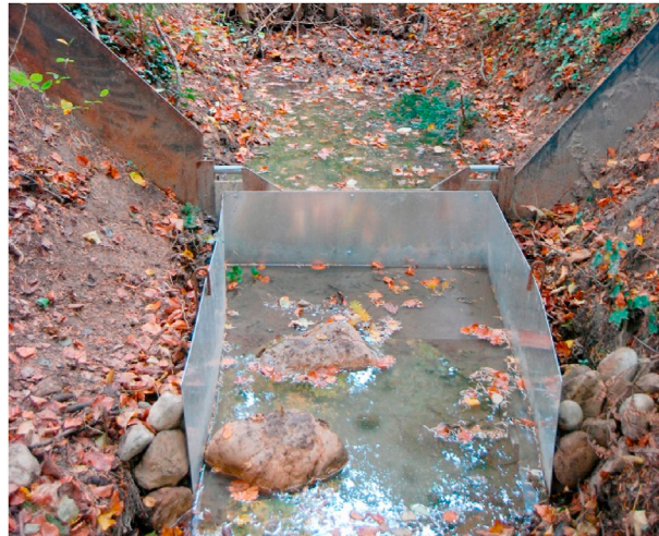
Fig. 7. Modified barrier with aluminium plates on both banks.
