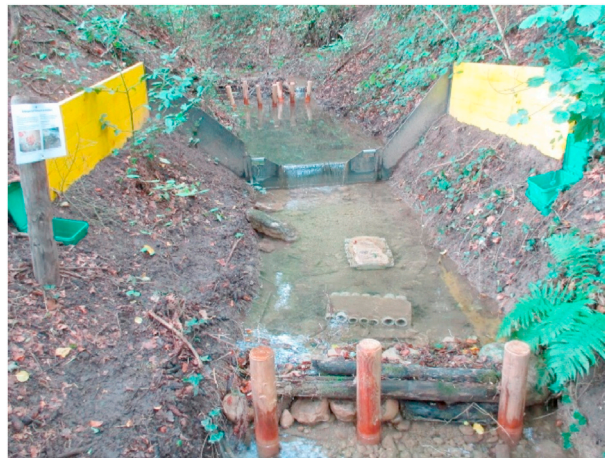
Fig. 5. Barrier with driftwood retention structure upstream and small dam further downstream.
