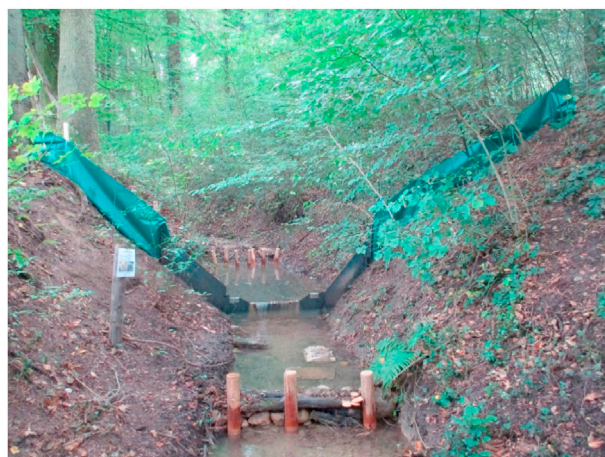
Fig. 6. Barrier including an extended land barrier on both banks.
