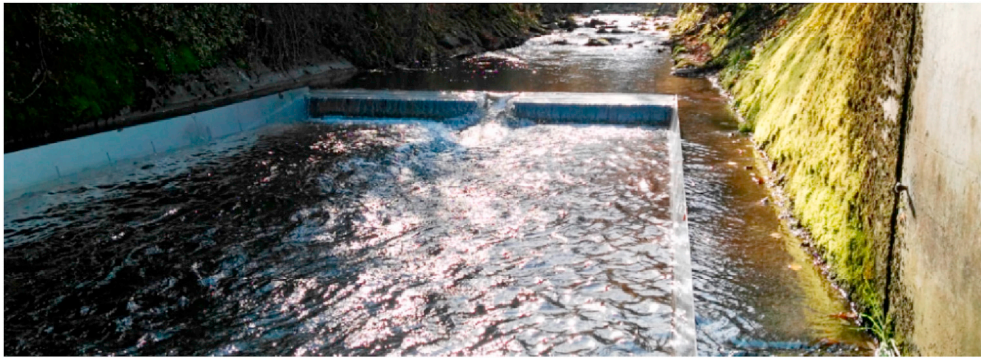
Fig. 10. Crayfish barrier in the Pfaffnern with a high-flow mid-section which is passable by fish.
