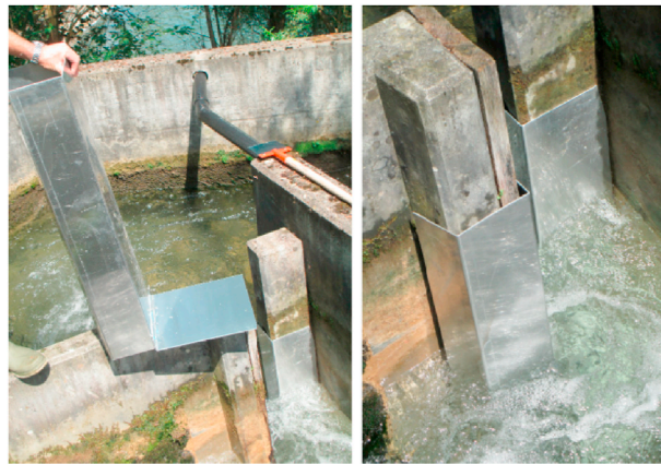
Fig. 2. Vertical-slot fish-pass with aluminium coating on the sections between the two pools.
