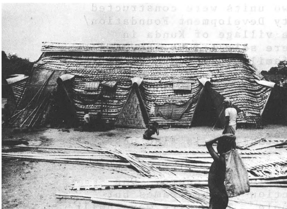
Figure 3. Photograph of the Mirpur Housing Project.
