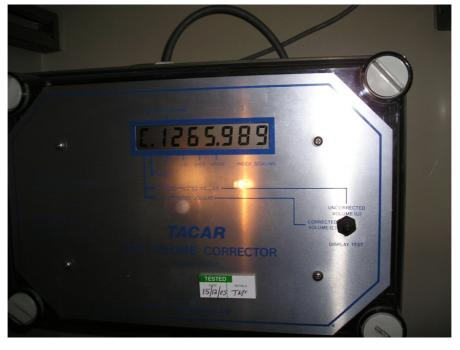
Fig. 1. The interface of the gas corrector meter in the input pipe to Edinburgh University's central area combined heat and power plant. Photograph courtesy David Somervell, Estates and Buildings, University of Edinburgh.
